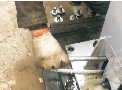
Fig7-2 The wire across the pillars back
