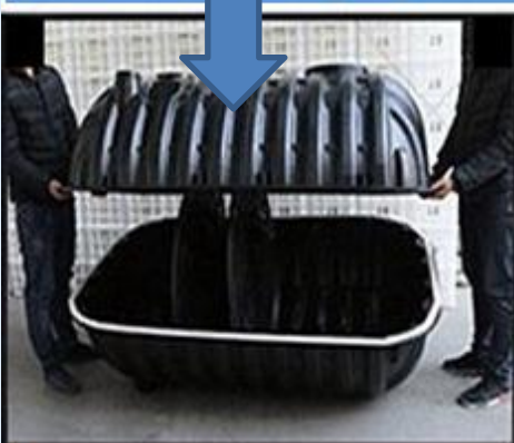
7. Install upper tank
