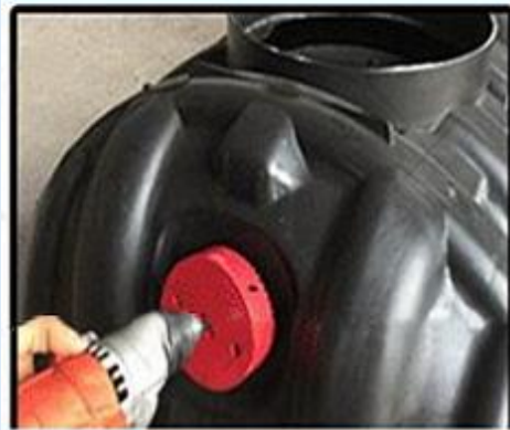
6. Open the water inlet/outlet hole, then install the sealing ring
